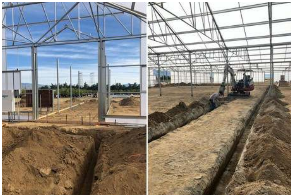
Building in progress!
