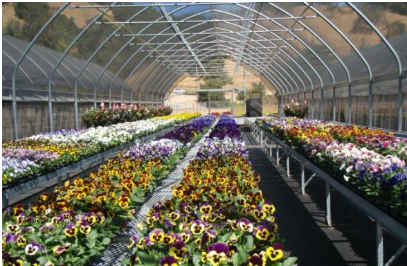
North Slope 24 with tie bars and webs covered in Shade Cloth. Note good interior clearance.
