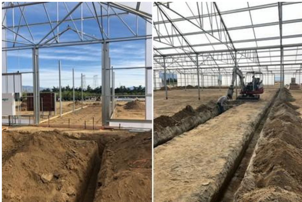
Building in progress!
